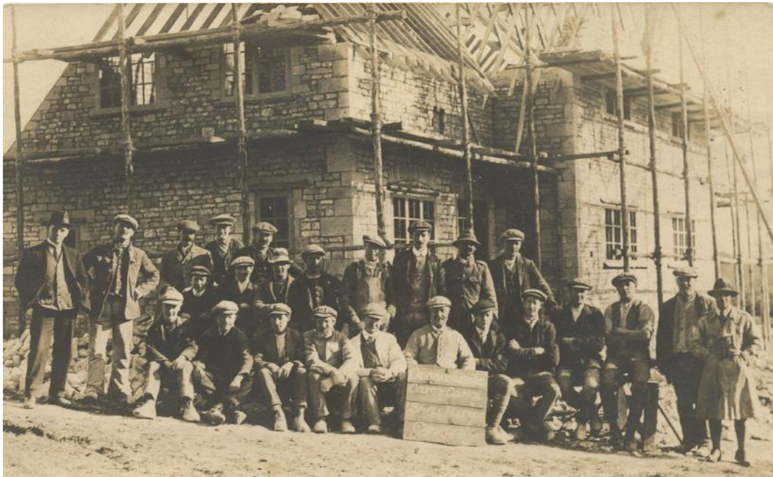
Working on the 'Homes for Heroes' in Aston Road
