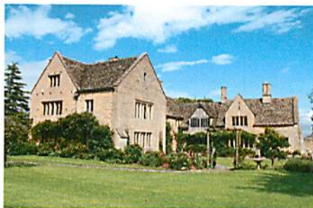
Fig 2. The West Wing in the foreground.
